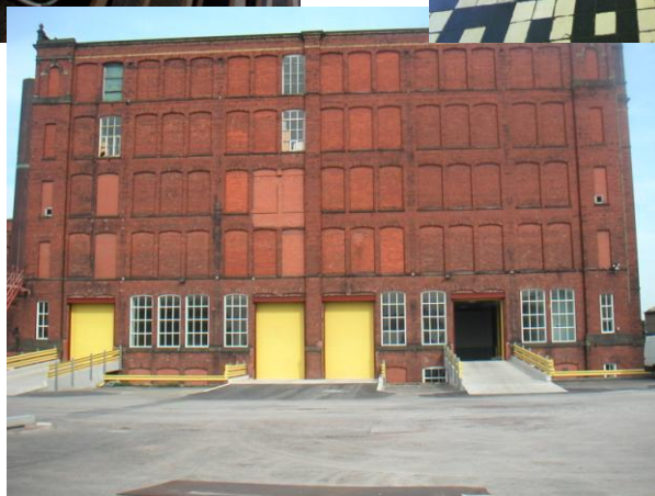
Loading Bays to Rear of Mill
